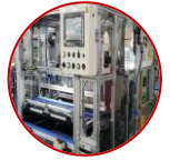
Automated assembly load line
